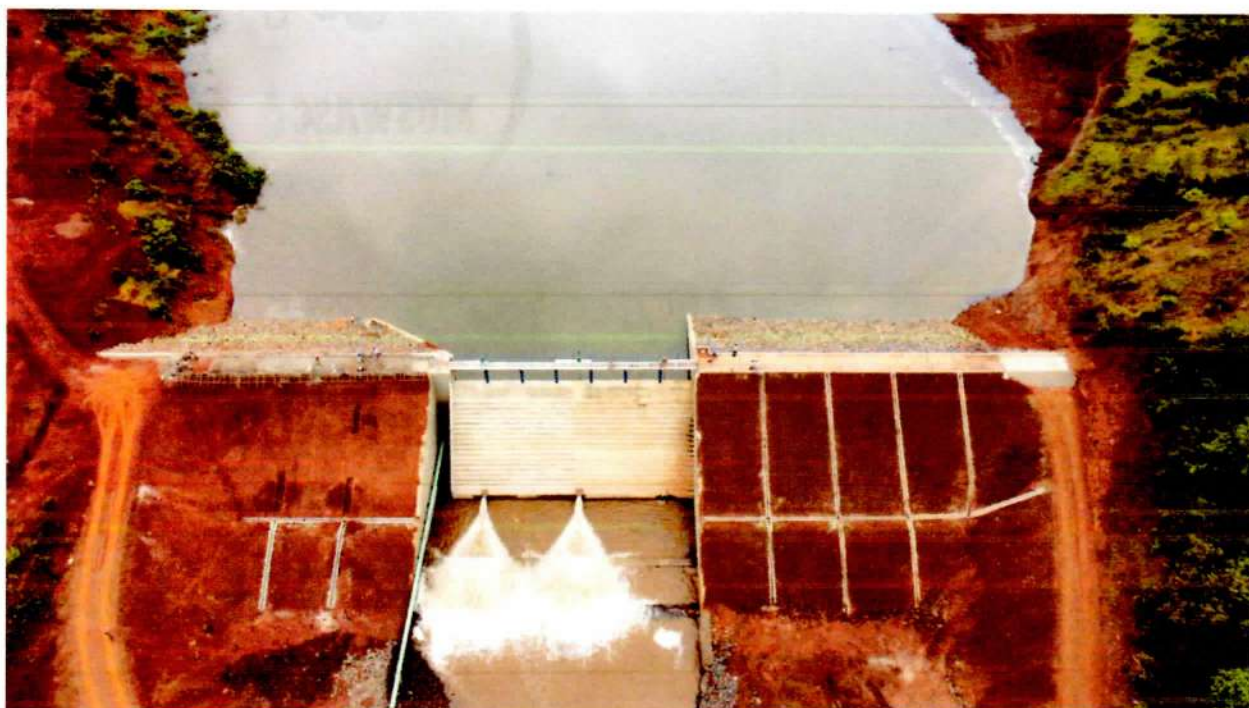
Figure 1 Maragua Bulk supply dam
